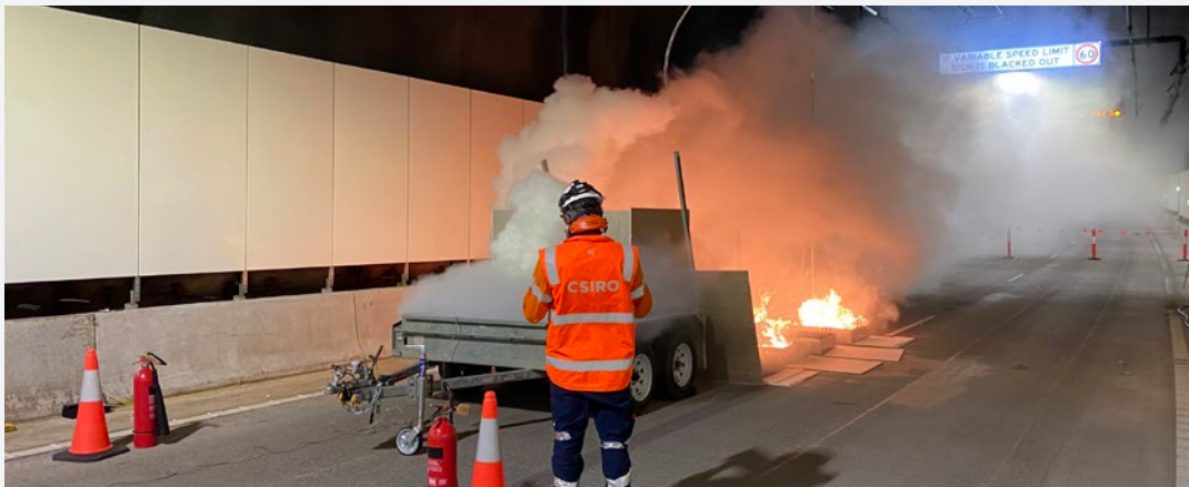
CSIRO fire safety engineering team conducts AS 4391 Hot Smoke Tests as part of commissioning requirements for major road and rail tunnel infrastructure across Australia.
