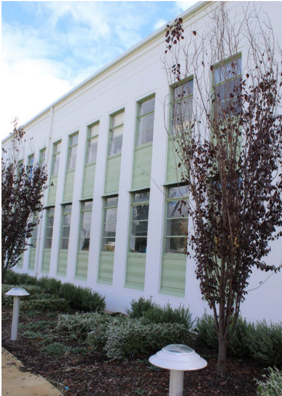
Figure 3.33 Detailed window treatment on the South Wing.
