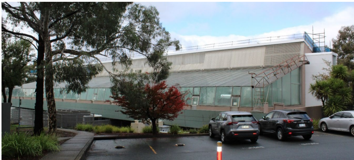
Figure 3.39 The northern elevation of the Phytotron and Phenomics Centre.
