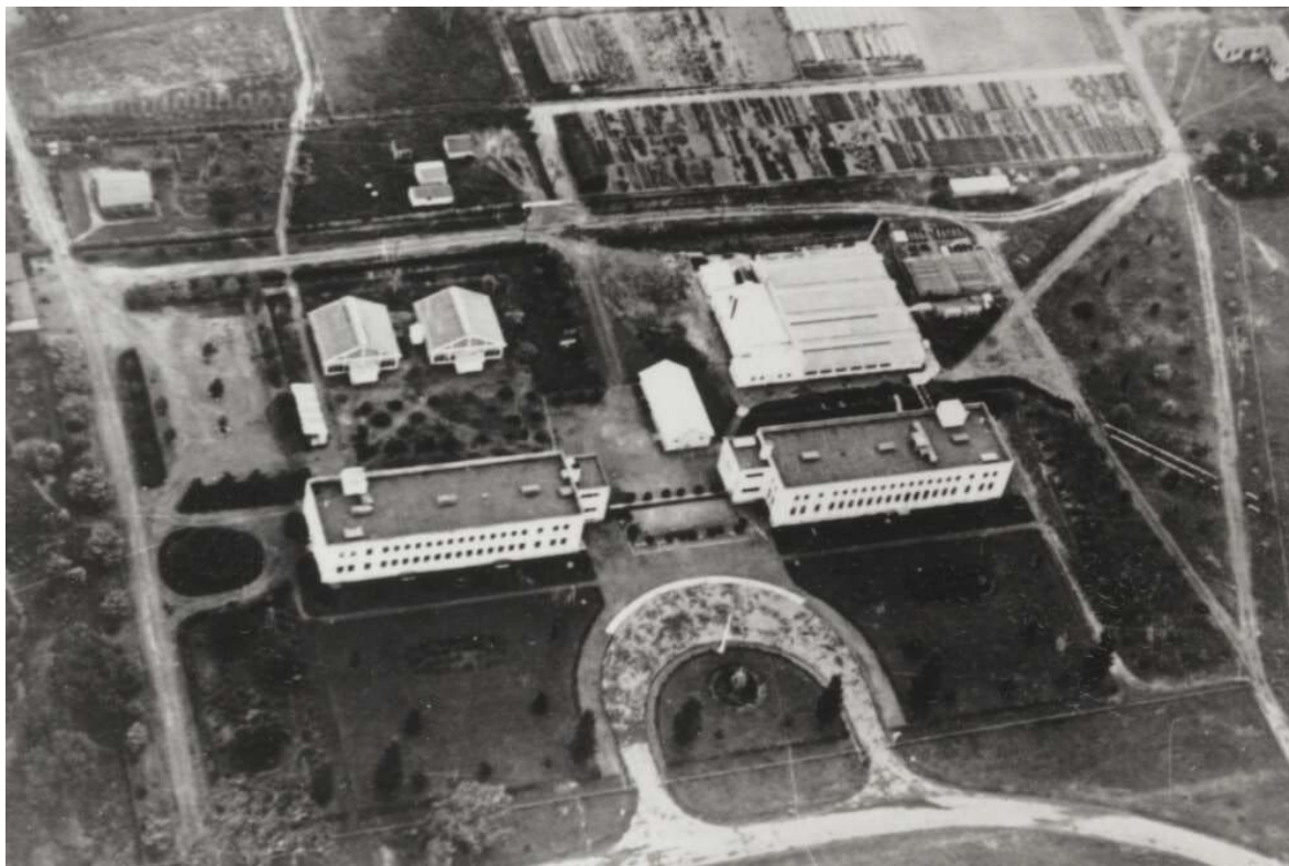
Figure 2.7 1938 aerial photograph showing the early period of construction, and experimental and research crops behind buildings and landscape planting. (Source: National Library of Australia, Bib ID 2254595)
