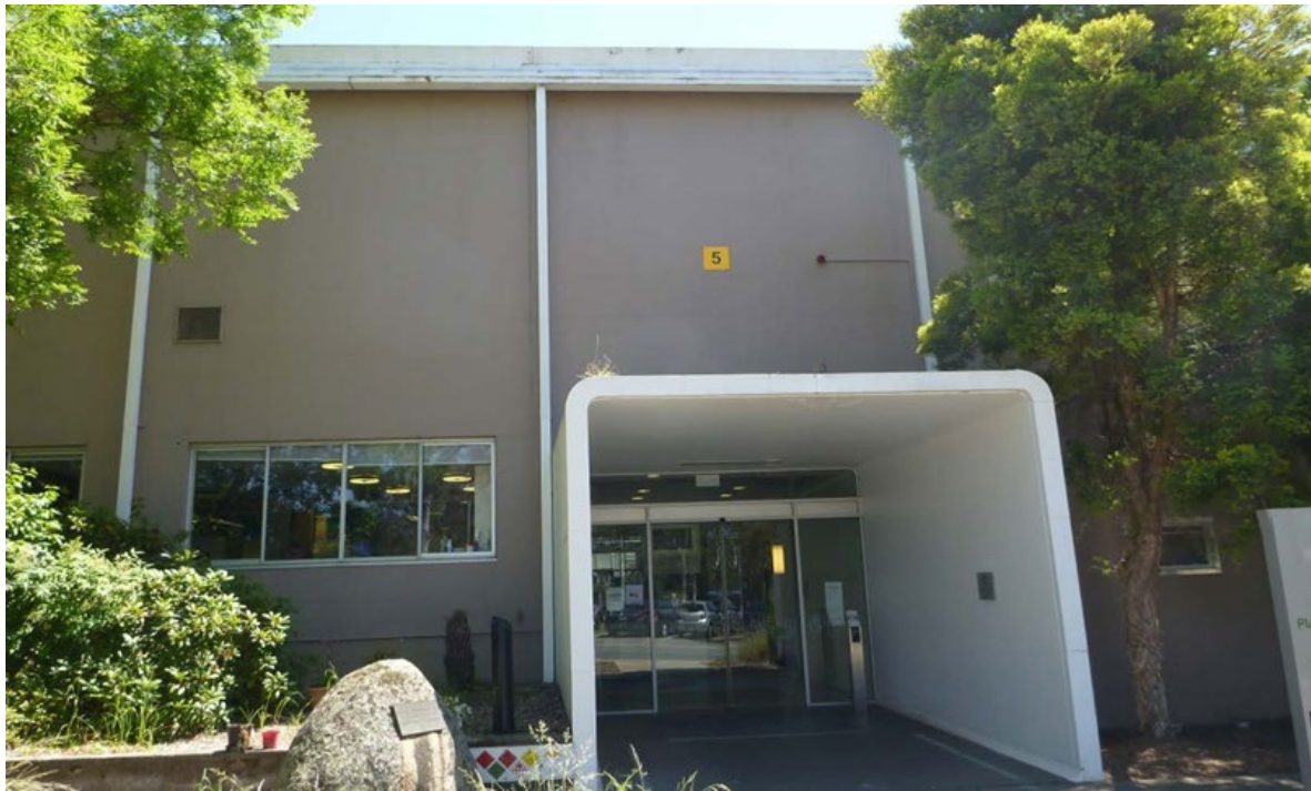
Figure 3.41 Main entrance to the Phytotron and Phenomics Centre, showing the deep, curved frame/portico. (Source: ERM 2015; a recent photograph was not possible due to scaffolding obscuring views)
