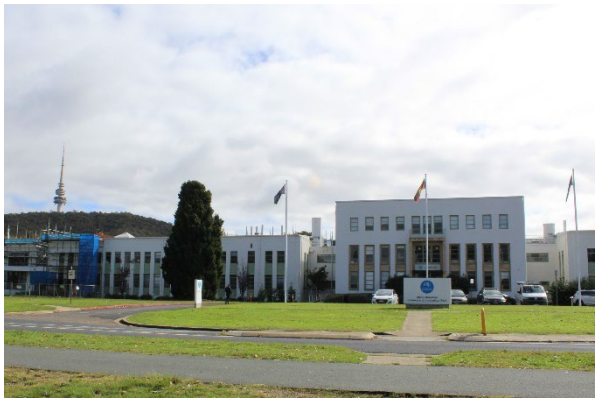
Figure 3.23 A photo from near Clunies Ross Street of the unimpeded view towards Foundation Building and Black Mountain beyond.
