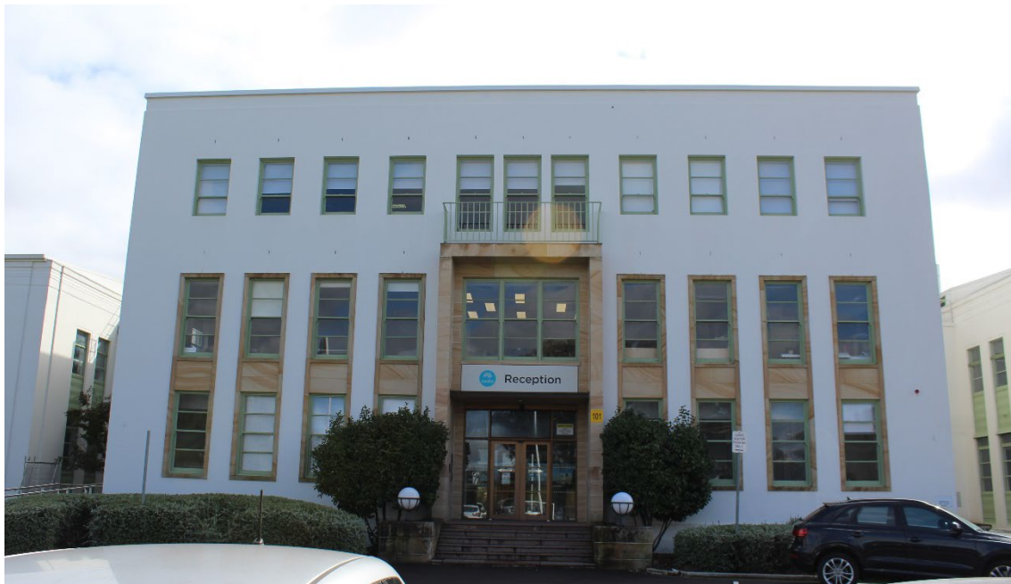
Figure 3.31 The façade of the Central Block. The sandstone portal, green painted timber windows with surrounding sandstone framing emphasises verticality—a characteristic of the inter-war Stripped Classical style of architecture.
