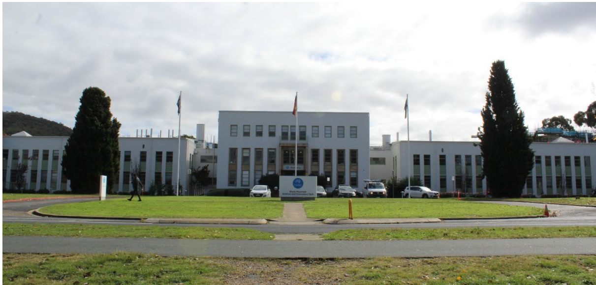
Figure 3.32 CSIRO Foundation Building (Building 101).
