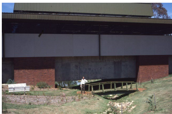
Figure 2.14 1980 photograph of Building 401C shortly after construction. The building was constructed over a small creek bed. (Source: https://csiropedia.csiro.au/csiro-computing-history-appendix-8-locations/ )
