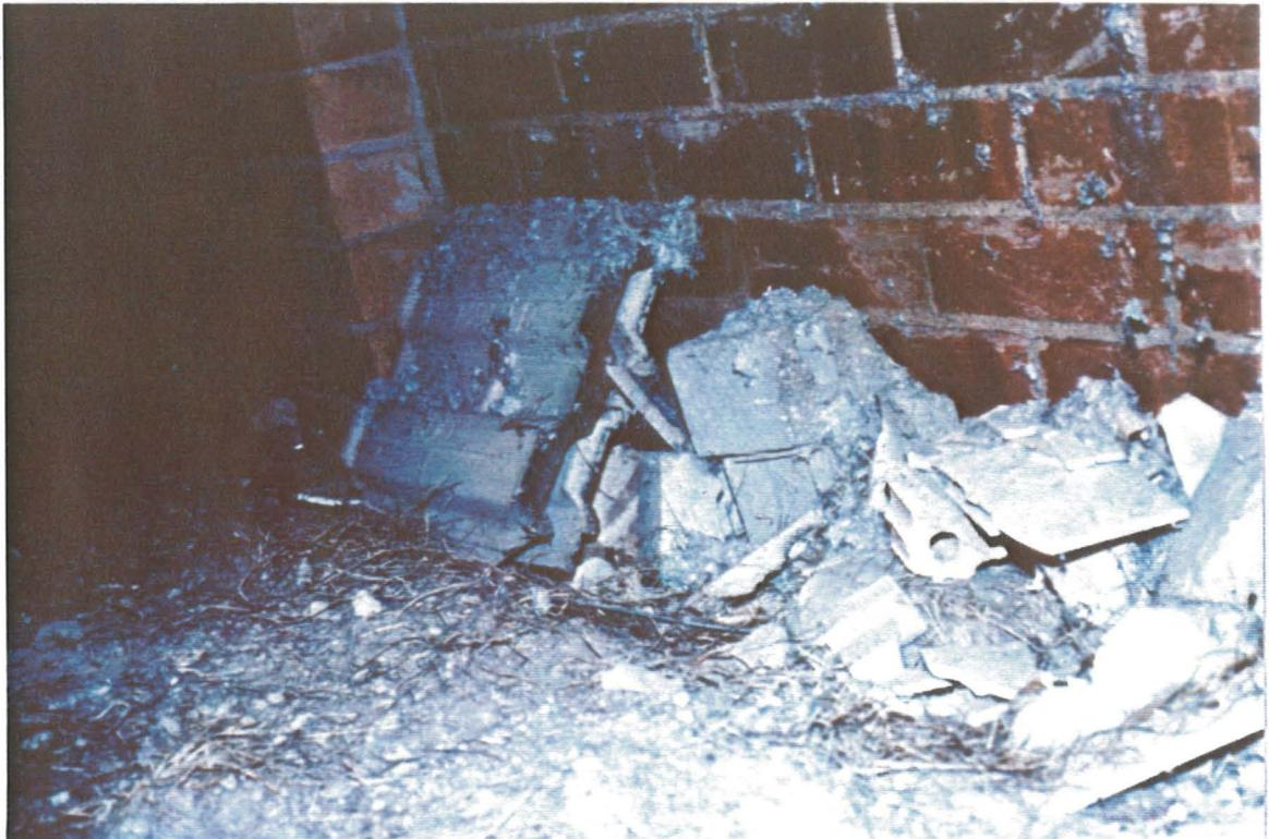
Figure 2. Bulk asbestos fluff residues in subfloor space of site 3.
