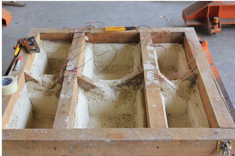
After Vermitex AF Installation
