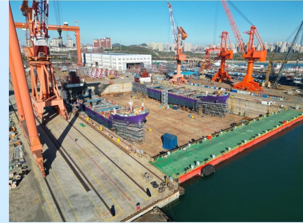
Figure 5: Northern Lights CO 2 carrier vessels under construction
