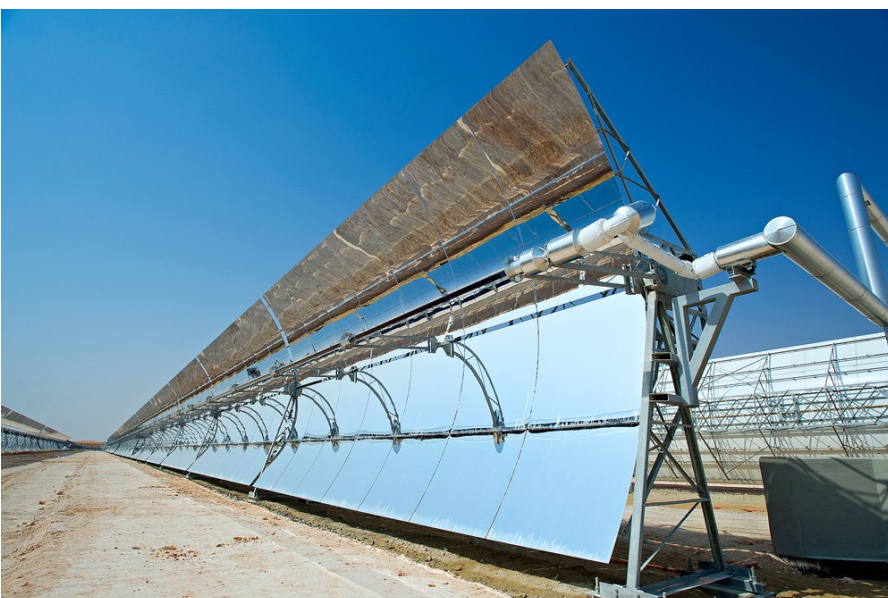
Figure 2 Parabolic trough solar collector at the Shams Solar Power Station in Abu Dhabi.
