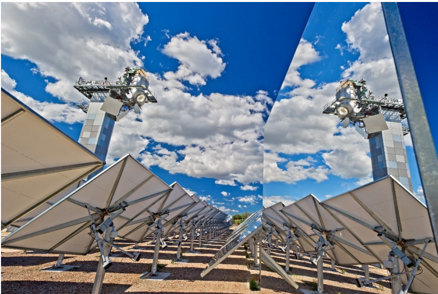
Figure 1 Solar thermal heliostat field and tower at CSIRO's solar thermal research facility in Newcastle.
