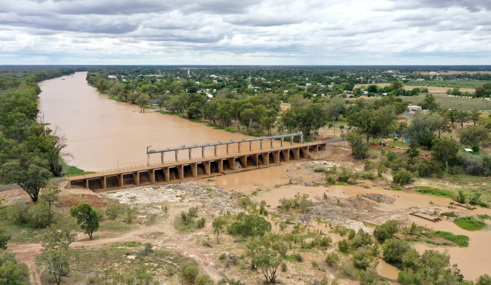
Jack Taylor Weir and the city of St George on the Condamine-Balonne River. Jack Taylor Weir is operated conjunctively with Beardmore Dam to supply water for irrigation, urban and industrial water users in St George.
