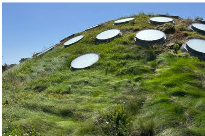
The amazing Living Roof of the California Academy of Sciences, featuring skylights for the exhibits below.
