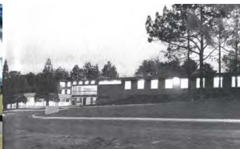
Former Forest Research Inst Bldg 1967
