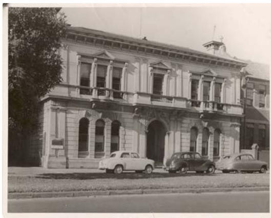
Figure 2 - Former CSIR Head Office, 314 Albert Street, Melbourne, Victoria
