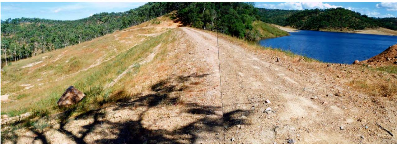
**Figure 3-5 Sharp-rock Dam embankment crest and batters**
