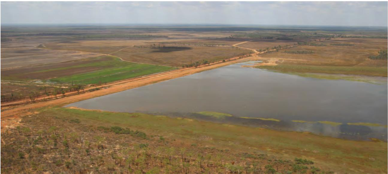
**Figure 1-2 Large farm-scale gully dam (~3.75 GL capacity) in Darwin catchments**
