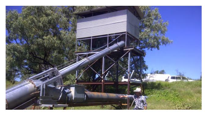
**Figure 3-2 Diesel powered axial-flow flood-harvesting pump in Flinders catchment, Queensland** Photo: CSIRO.
