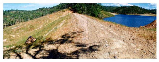
**Figure 3-5 Sharp-rock Dam embankment crest and batters** Photo: North Australia Water Strategies
