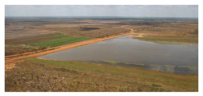
**Figure 1-2 Large farm—scale gully dam (~3.75 GL capacity) in Darwin catchments** Photo: CSIRO.
